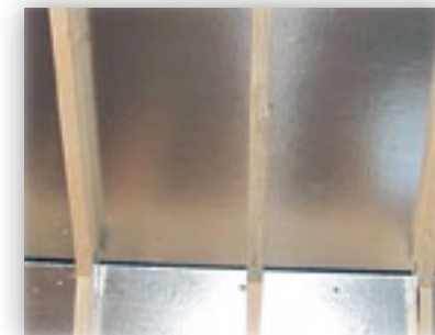
Radiant Barrier Thermostat R.B. (Roof)—$.75 sq. ft. SilverTech R.B. (Walls)—$1.50 sq. ft.
